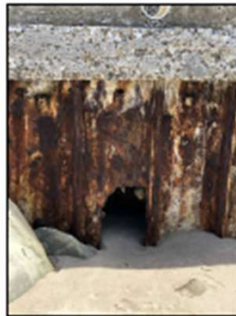
A1 EXISTING STEEL SHEET PILE (CUT OFF AND REMOVE UPPER 1 FT AND REPAIR HOLES)
