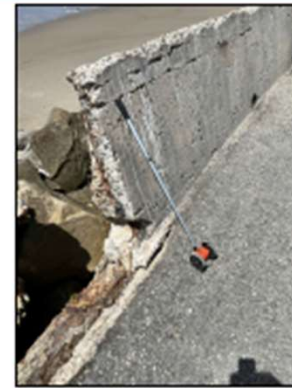
D4 EXISTING CONC PARAPET WALL (DEMOLISH AND REMOVE)
