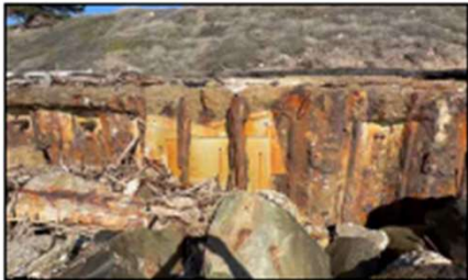
A1 EXISTING STEEL SHEET PILE (CUT OFF AND REMOVE UPPER 1 FT AND REPAIR HOLES)
